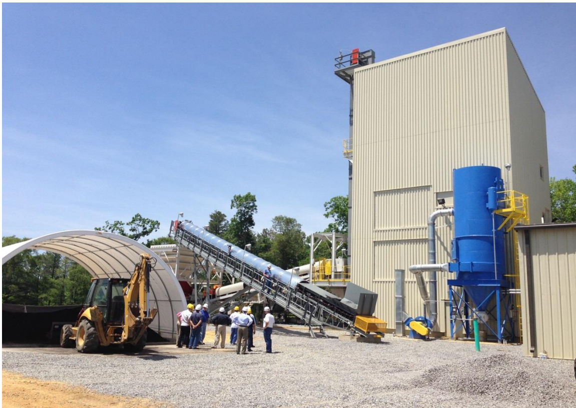
Image 1: The TMS "Generation II" Commercial Demonstration Facility
