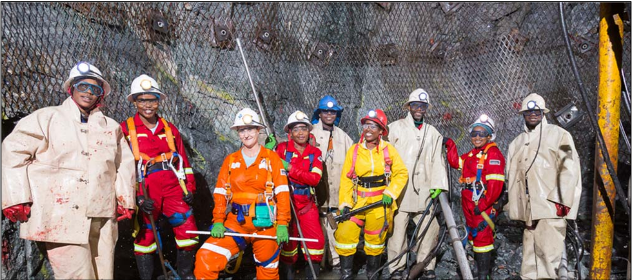
Figure 1: Members of Platreef’s shaft-sinking team in Shaft 1 at a depth of 500 metres below surface, more than halfway to the planned final depth of 980 metres.
