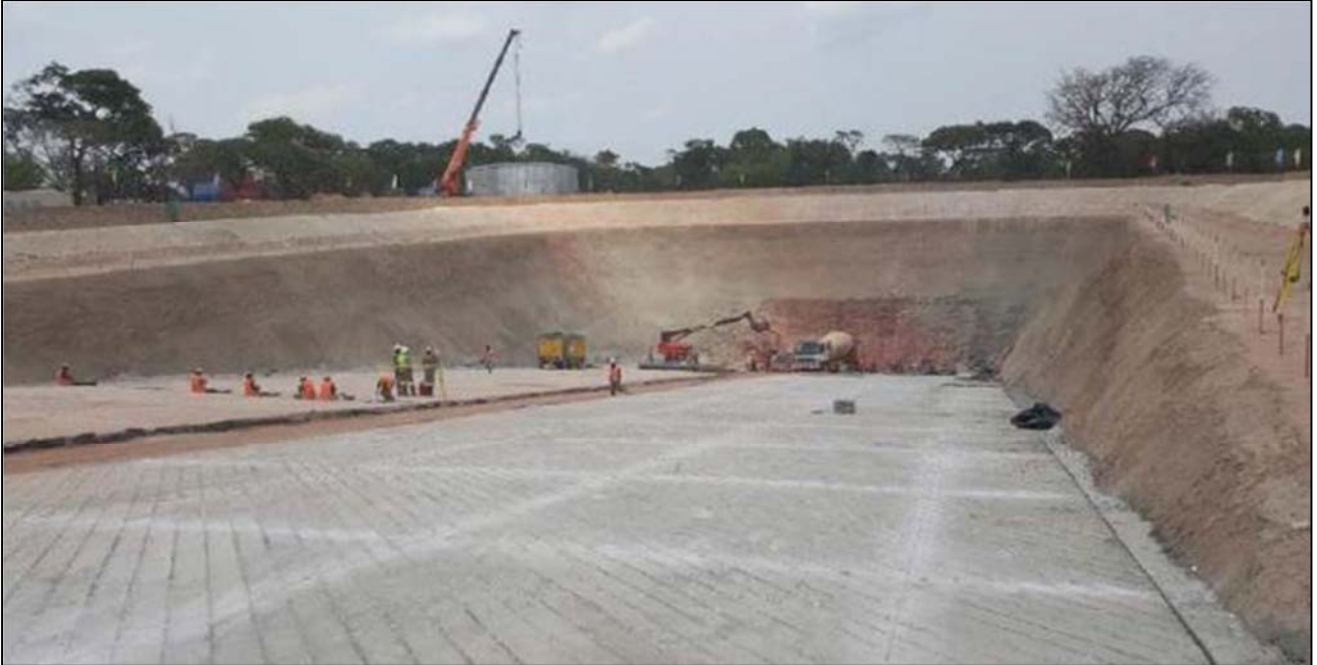
Figure 9 and 10: The Kakula box cut was completed on October 26, 2017. The first blast for the access declines is scheduled for mid-November 2017.
